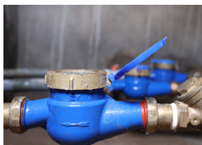
Bulk meters installed to monitor NRW on the Ngabwe-Ryarubondo-Kabuga, Nyamagabe District.
