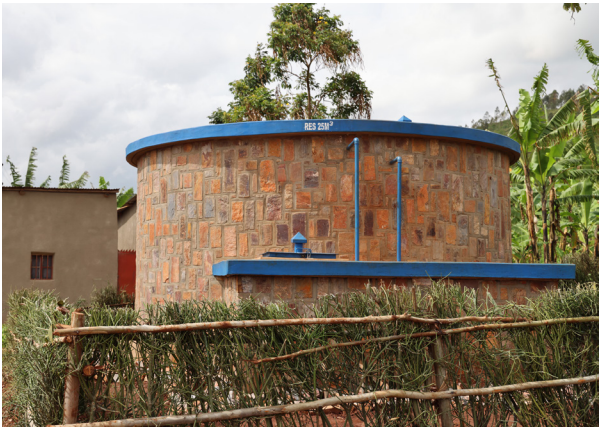
A 25 m3 reservoir was rehabilitated.
